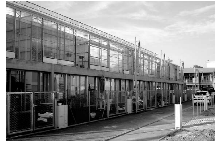
Above: Nemausus 1 in Nîmes, France 1988, designed by Jean Nouvel. Photo by Shinkenchiku-sha. Below: Mulhouse 2004, designed by Lacaton & Vassal. Photo courtesy of Lacaton & Vassal.
